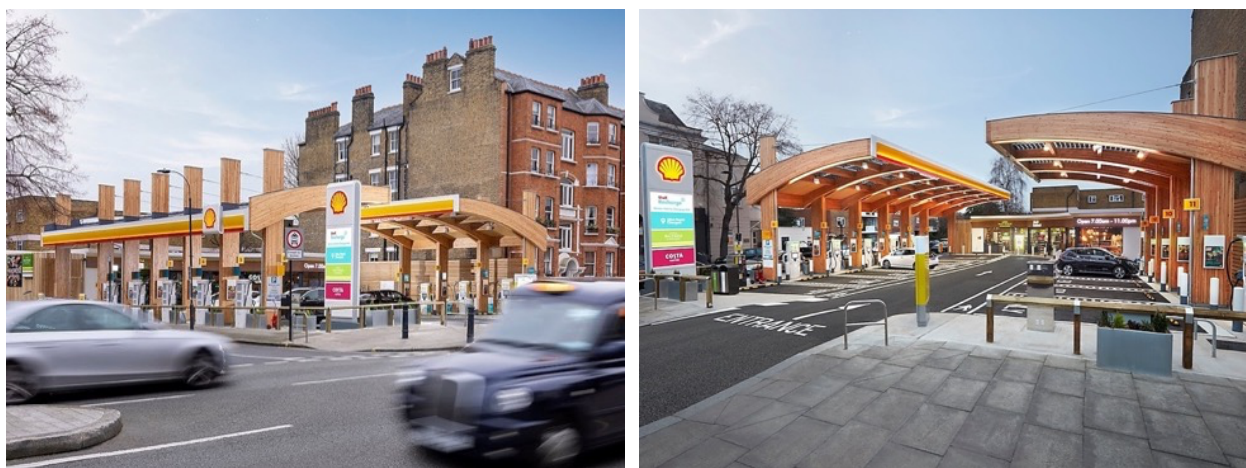
Figure 7 EV charging station similar to a petrol station (Fulham, London)
