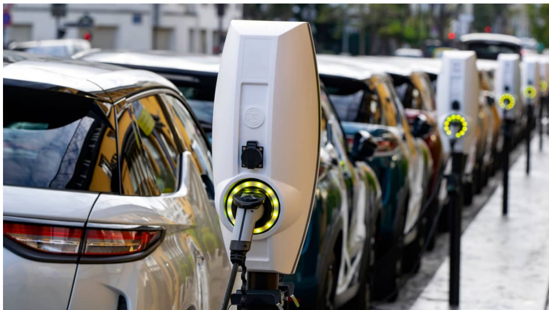
Figure 6 Example of multiple on-street Level 2 charge points for longer term stay periods
