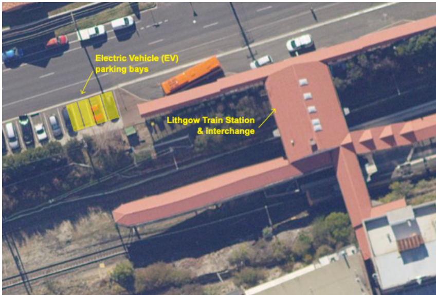
Figure 10 Parking bays to west of entry to Lithgow Rail Station from Railway Parade
