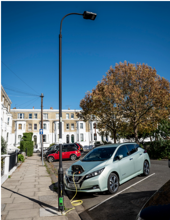
Figure 47 Lamp post charging, London
