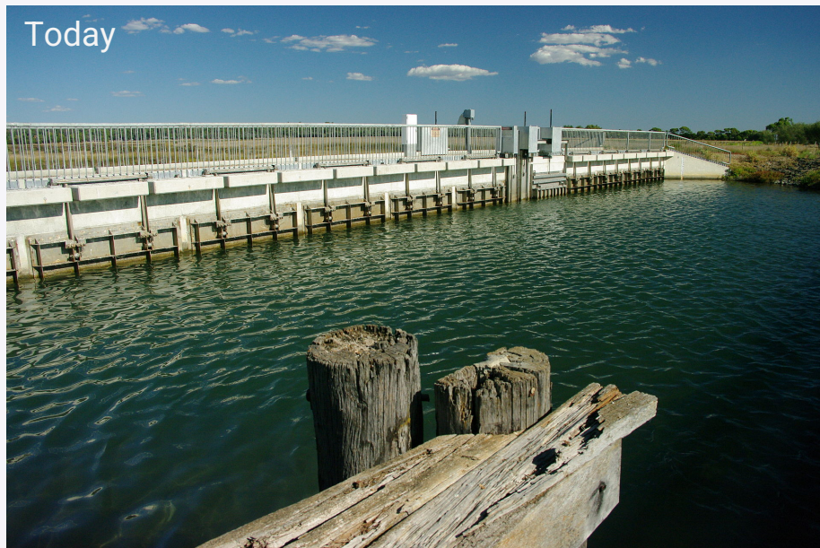
Wonnerup floodgates – Vasse River, WA
