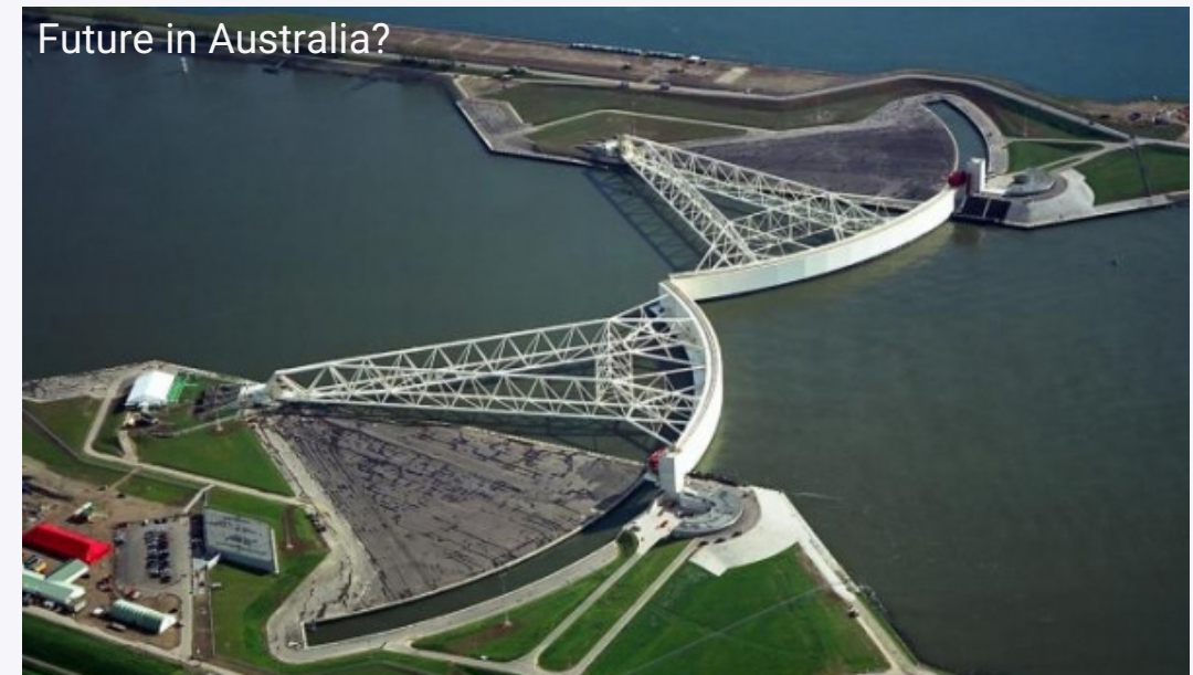
Maeslant barrier, Rotterdam, The Netherlands
