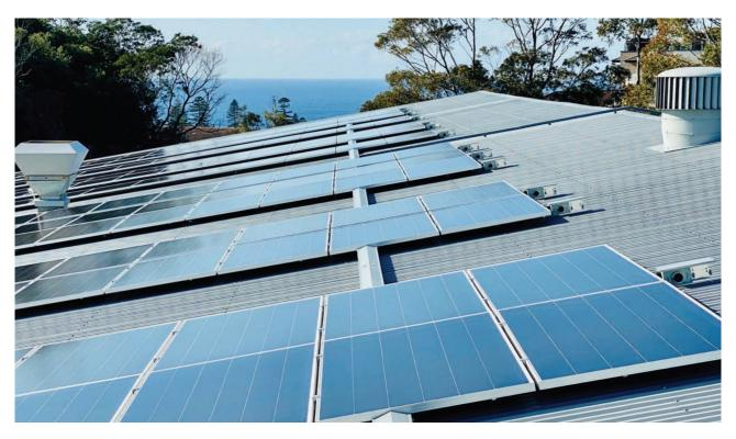
Kiama Leisure Centre - 99.6kW Photovoltaic system reduces energy consumption on site by 30% annually.
