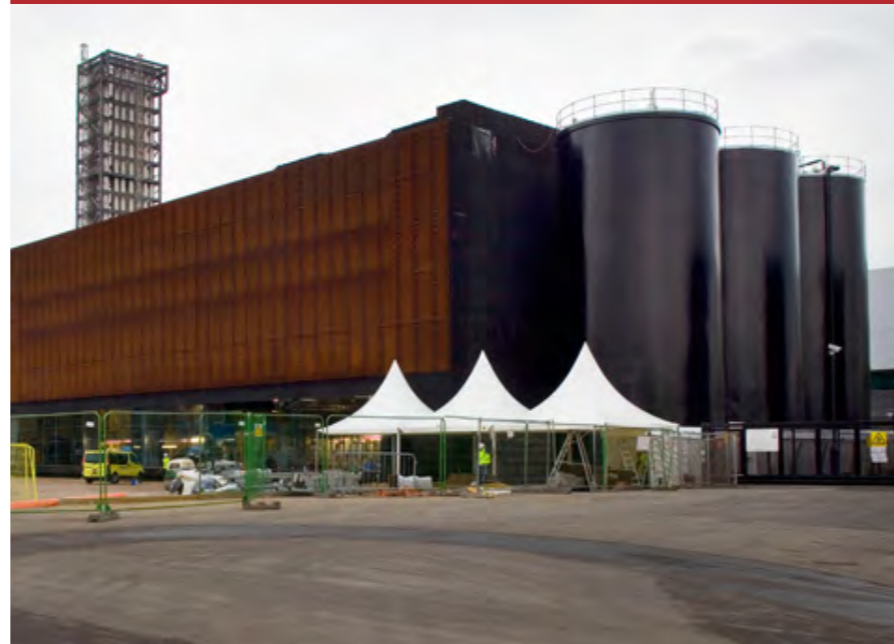
FIGURE 103: RENEWABLE FUELLED TRIGENERATION ENERGY CENTRE, KINGS YARD, OLYMPIC PARK, LONDON, UK
