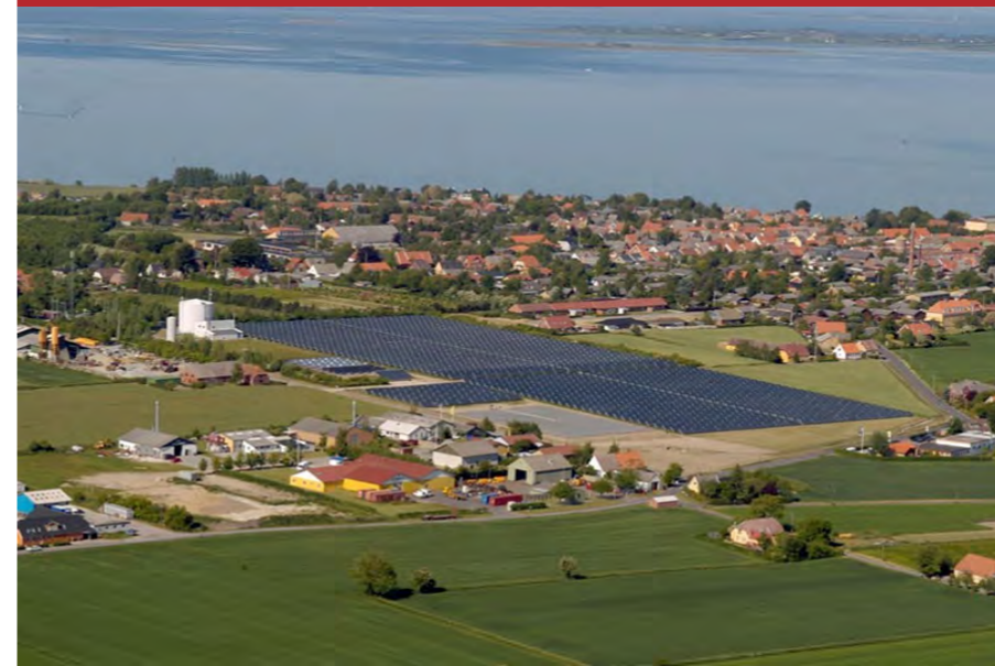
FIGURE 63: SOLAR FIELD SUPPLYING MARSTAL DISTRICT HEATING SYSTEM, DENMARK SOURCE: DENMARK.DK
