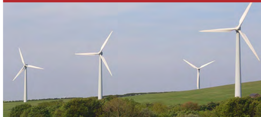
FIGURE 89: BAYWIND ENERGY – FURNESS WIND FARM, HARLOCK HILL, CUMBRIA, UK SOURCE: RENEWS
