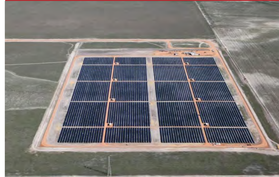
FIGURE 68: GREENOUGH RIVER SOLAR PV FARM, WESTERN AUSTRALIA SOURCE: GREENOUGH RIVER SOLAR FARM
