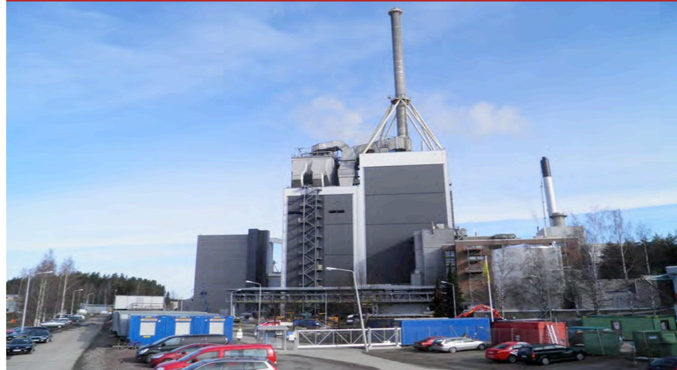
FIGURE 84: KYLMÄJÄRVI 2 MUNICIPAL WASTE GASIFICATION RENEWABLE GAS FUELLED COGENERATION NETWORK, LAHTI, FINLAND SOURCE: LAHTI ENERGIA
