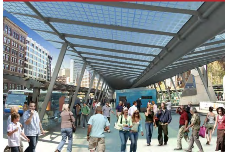
FIGURE 61: PROPOSED GLASS/GLASS/PV SOLAR CANOPY AT RAILWAY SQUARE BUS INTERCHANGE SOURCE: CITY OF SYDNEY
