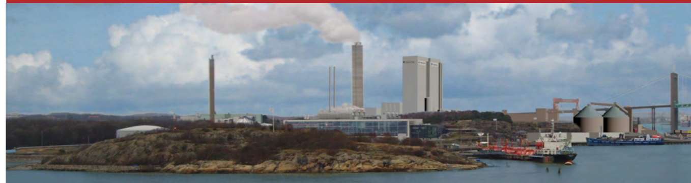
FIGURE 83: GOBIGAS BIOMASS GASIFICATION RENEWABLE GAS GRID INJECTION – PHASES 1 AND 2, GOTHENBURG, SWEDEN SOURCE: GOTEBURG ENERGI
